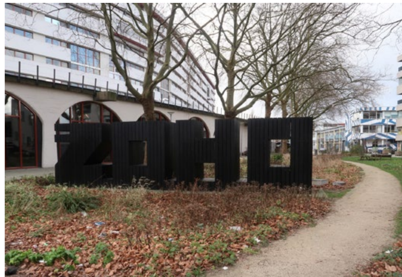
Image 11: Example of waterstorage measurement by Rotterdams Weerwoord in ZOHO; the water is collected from the Hogbogen into the letters (Robert van Overveld, taken on January 15, 2023)
