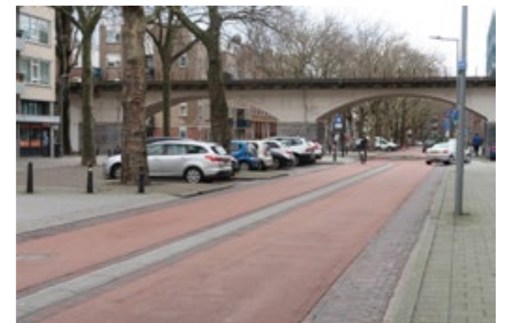
Image 97: Example of cyclist street with a small path for cars (Robert van Overveld, taken on 15 January, 2023)
