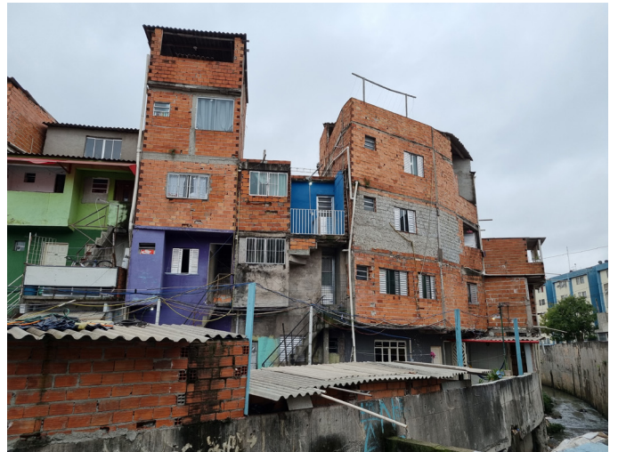
Figure 9. Irregular settlements in Heliópolis.
