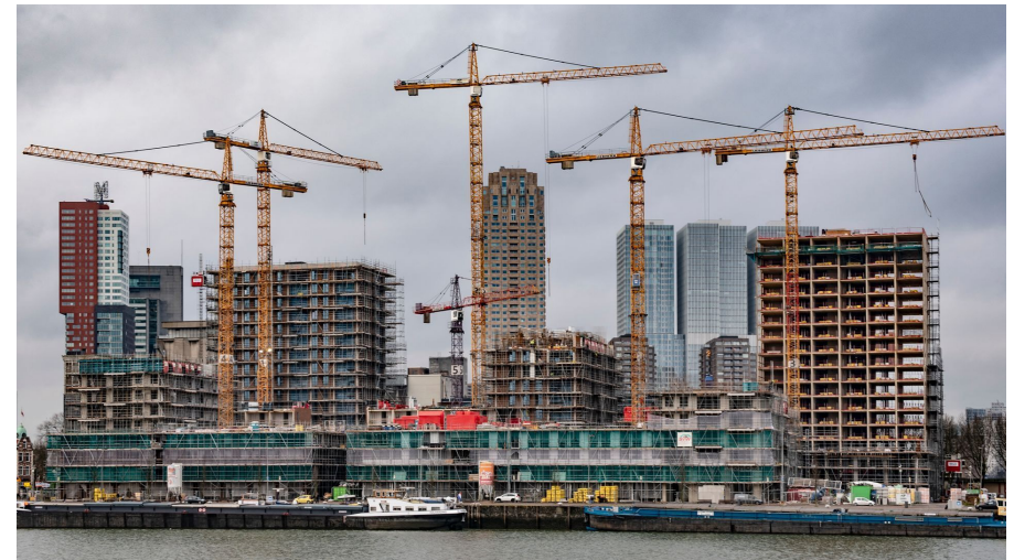
Figure 1 Cranes in the sky as Rotterdam's skyline builds upwards Rijnmond & NOS, 2022
