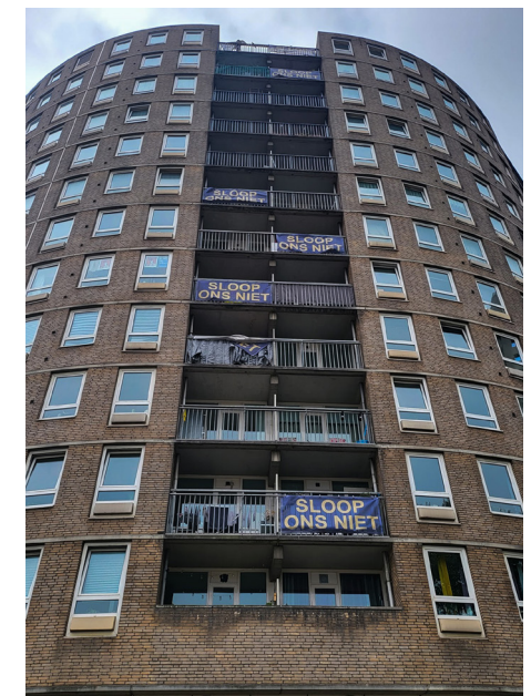
Figure 2 Protest banners on the facade of a Rotterdam residential block exclaiming "Don't demolish us"
