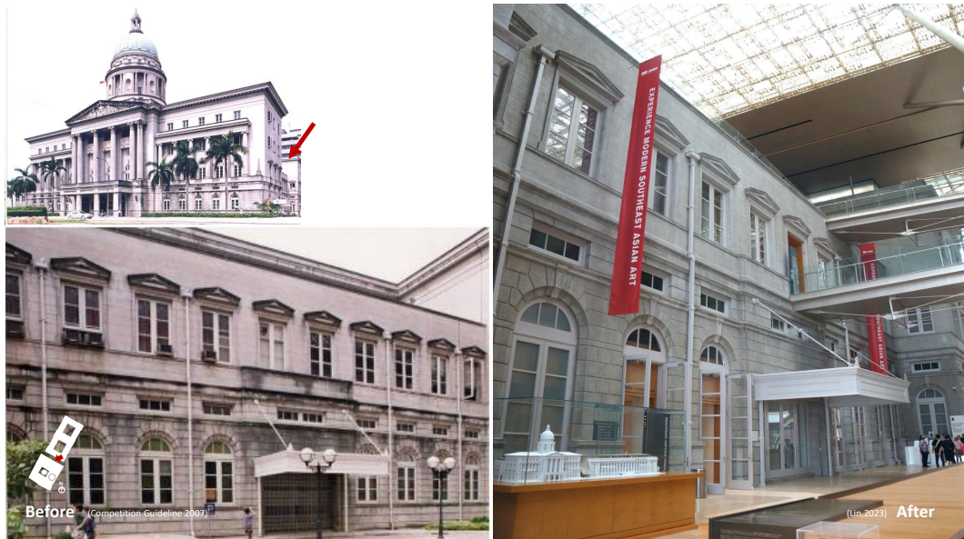
FIG. APP. 2.6. The entrance for the Chief Justice at the former Supreme Court. The Chief Justice used to take a private elevator and arrive directly at his office above. After (left): After the intervention, the entrance is closed and replaced by two side doors to access the exhibition spaces. A new bridge was added to the new gate by enlarging the original window opening. This intervention was considered controversial due to the interruption of the original spatial experiences of the Chief Justice.
