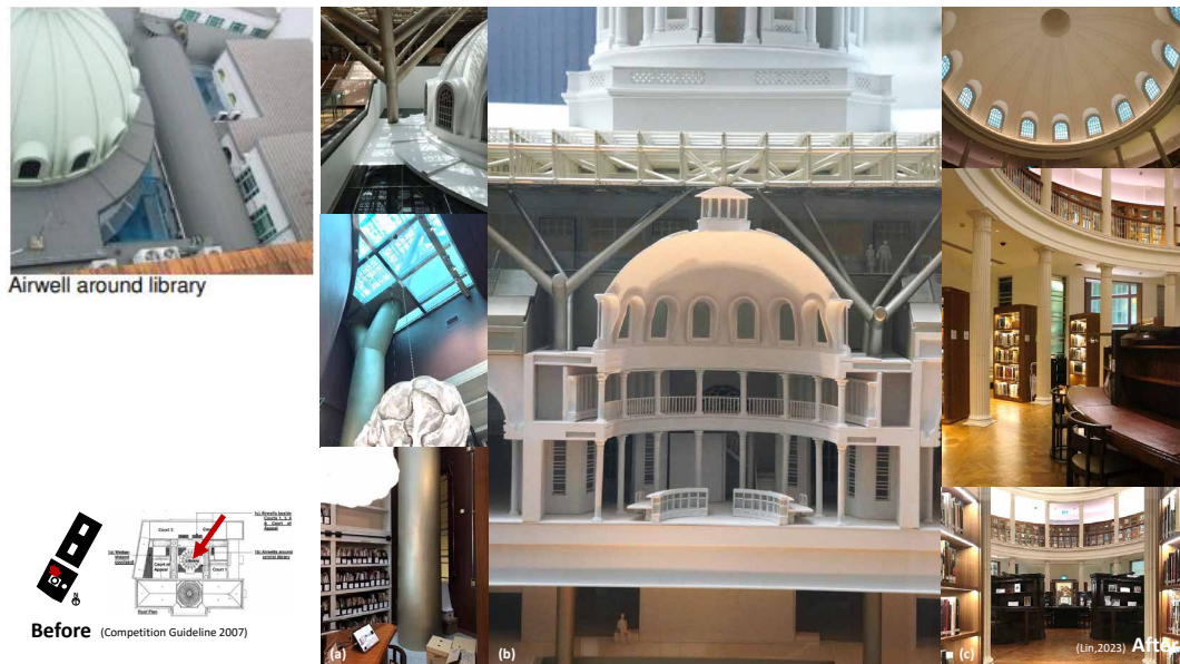
FIG. APP. 2.12. A close look at the interventions in the library under the “second dome”. (a) new tree-like columns were added to support the new roof. The interior of the library, including the wooden furniture, has been restored. This space is now open for visitors, especially for checking and reading law-related publications.
