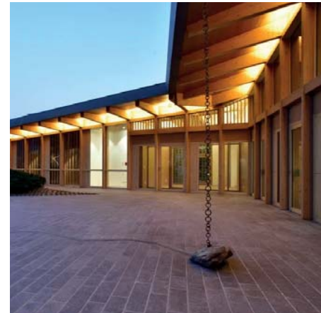
Rainwater Harvest System
