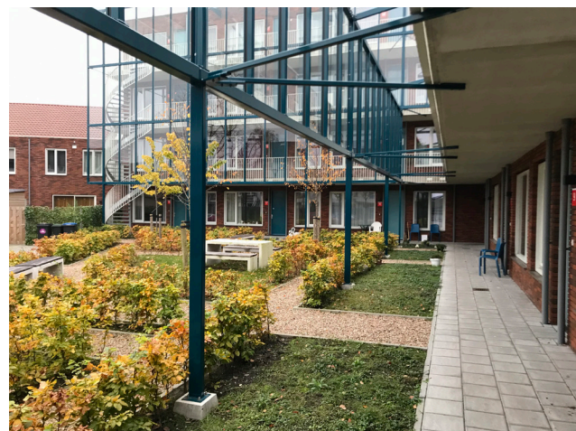
Photo 3: Gallery access to the individual apartments.
