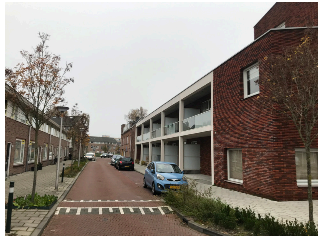
Photo 1: Road towards the housing facility (on the right).
