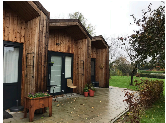
Photo 13: Outdoor access to the individual units.
