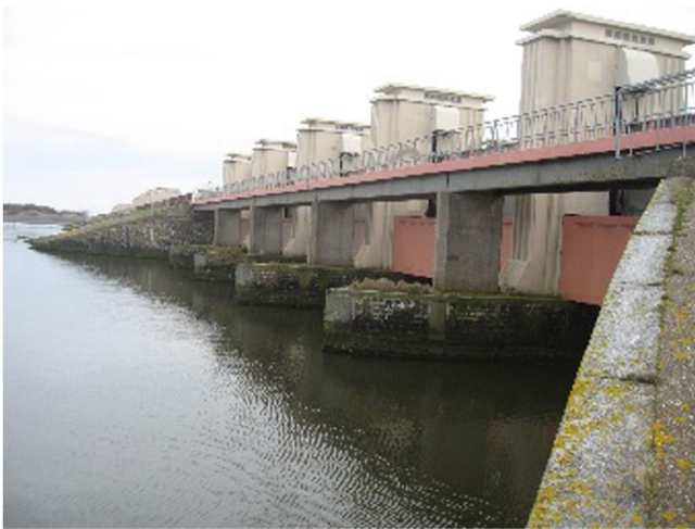
Figure 16. Discharge sluice in the closure dam (built 1932; source: beeldbank RWS).
