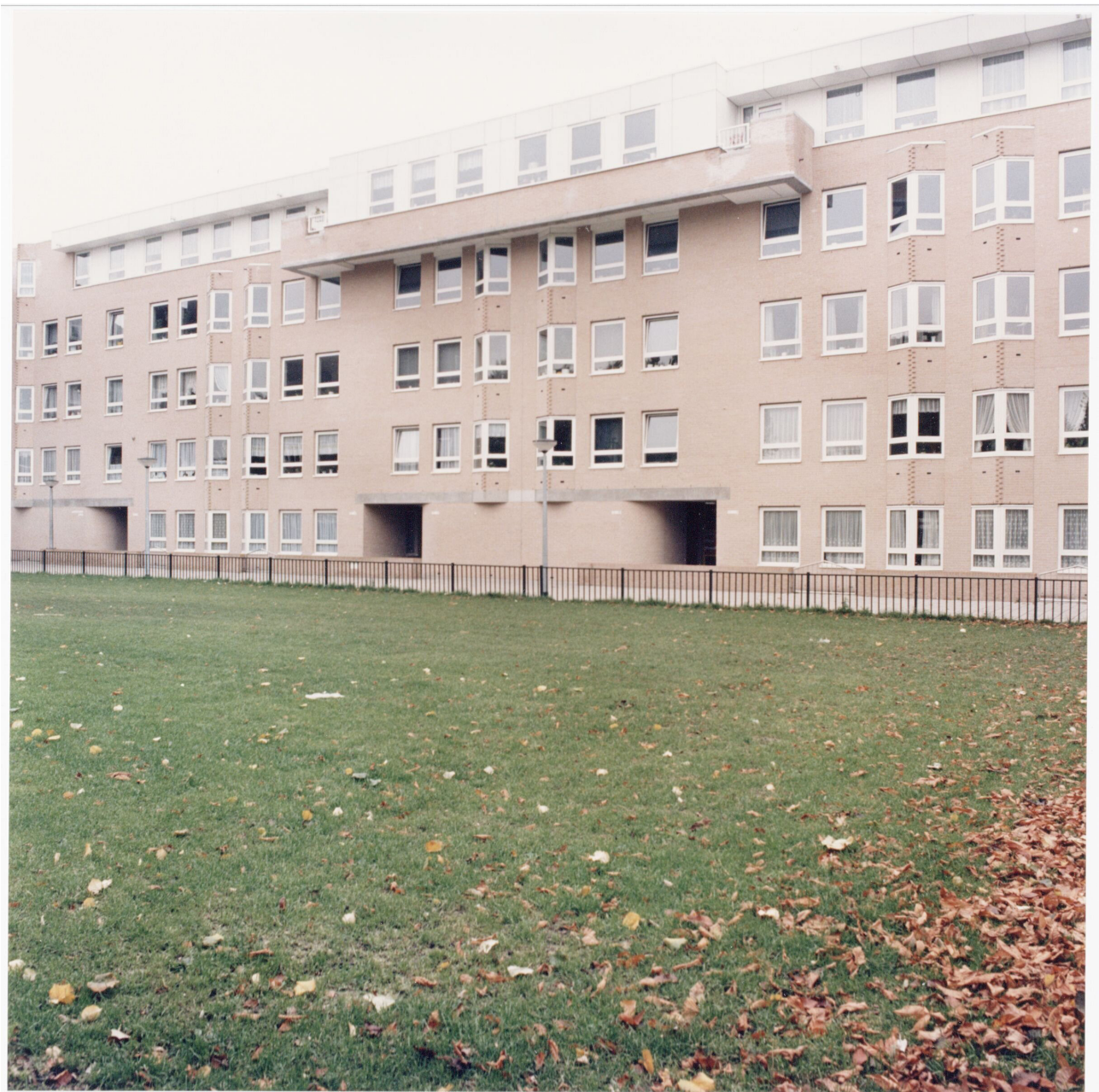
Fig. 12 Apartment complex Borssenburgplein (Unknown Photographer, n.d.).
