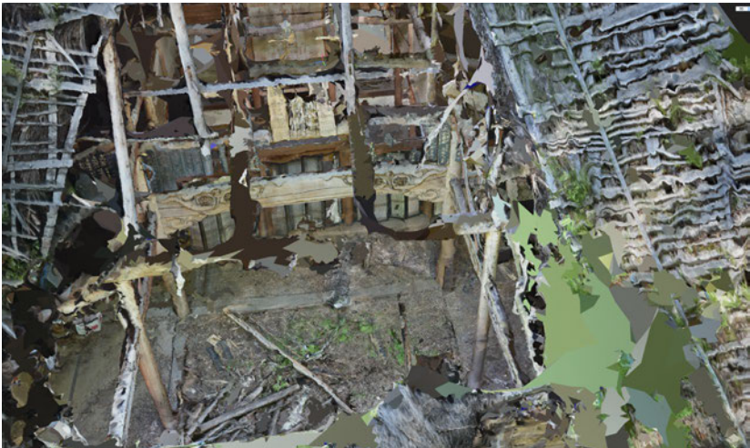
Figure 21-23 Mesh reconstructions of the Anyoji photogrammetry model
