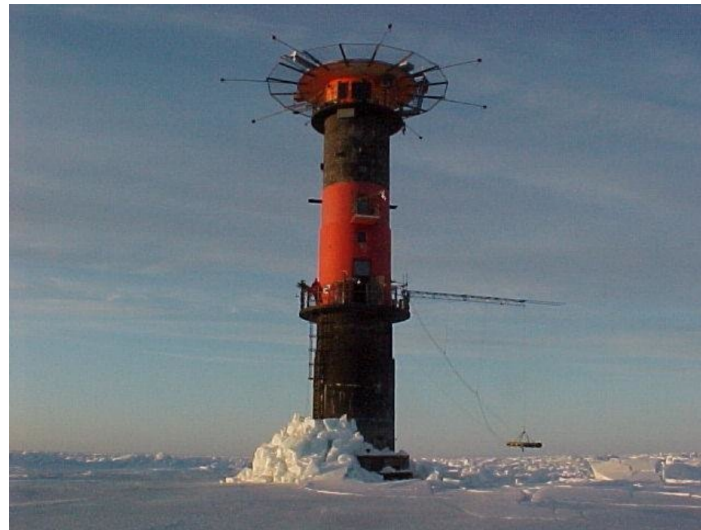
Figure 4-1: Photograph of the Norströmsgrund Lighthouse with a rubble pile after crushing failure of drifting level ice (Photo by Kari Kolari, VTT).
