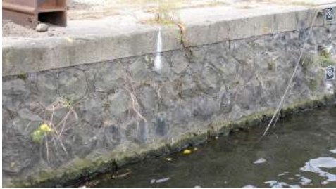
(a) Basalt quay wall, which has a good texture for finding features.
