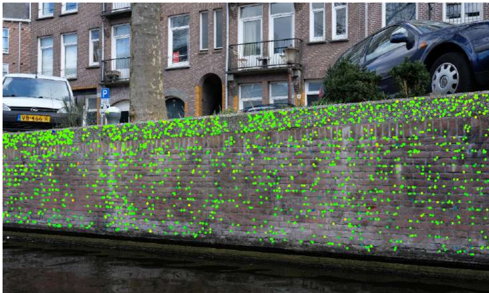
Figure 5.2: Deformation point visualization where the deformation points are projected onto the images used in the deformation analysis. In this image the deformation points are coloured to the deformation size in Y direction (into the quay wall).
