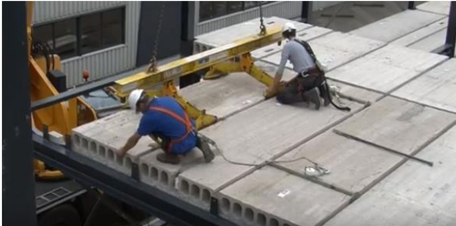
Figure 4.2: Circular hollow-core slab floor
