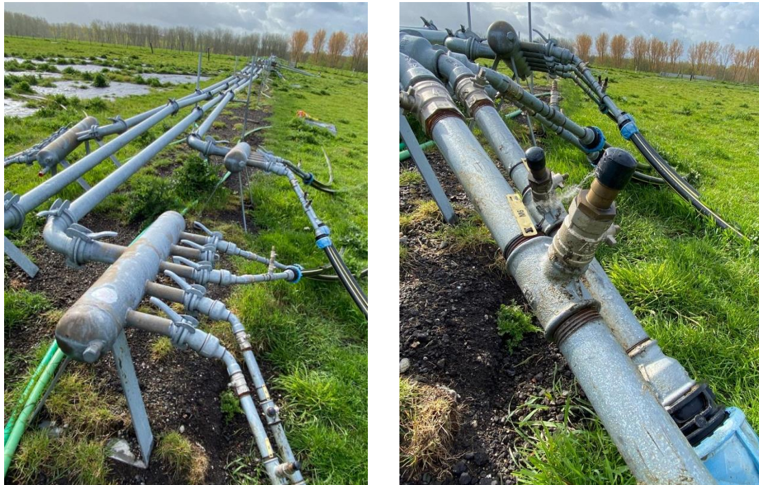
Figure 5.2: Divider system (left) and access point to the tubing (right)
