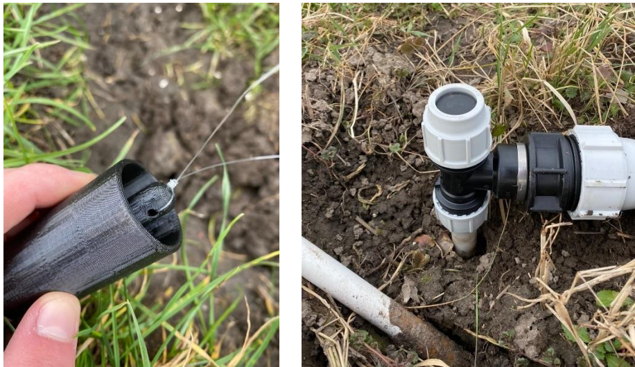
Figure 5.7: 3D printed connection piece (left) and closed well after installation (right)
