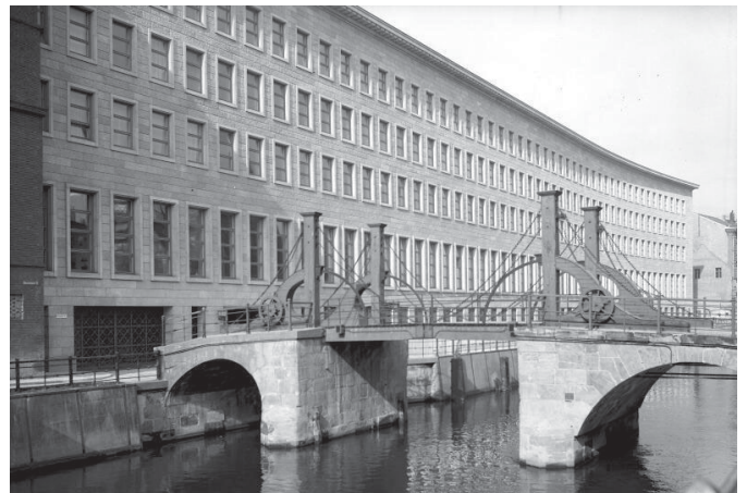
Fig 18: Backside of the Reichsbank and the Jungfernbrücke (Unknown, 1930-1940)
