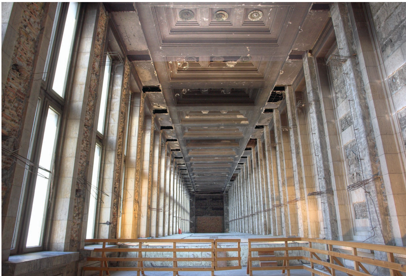
Fig 43: The unused upper part of the entrance hall created by the installation of the intermediate floor (Wikimedia, 2008)
