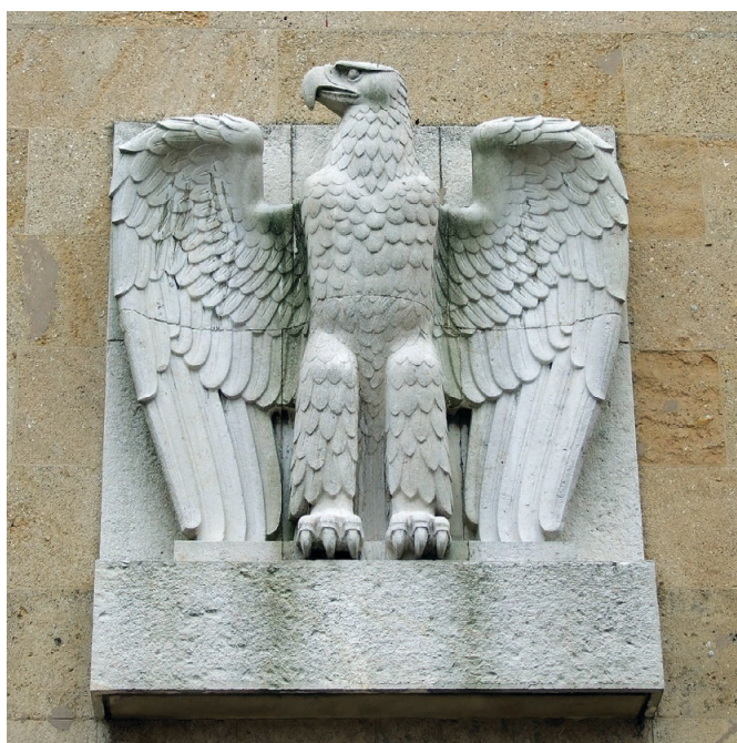
Fig 29: Nazi eagles such as these are still present on the façade of Tempelhof Airport, the Swastika underneath them has been removed (Joe, 2008)
