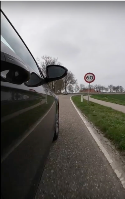
(c) Speed limit signs placed too late
