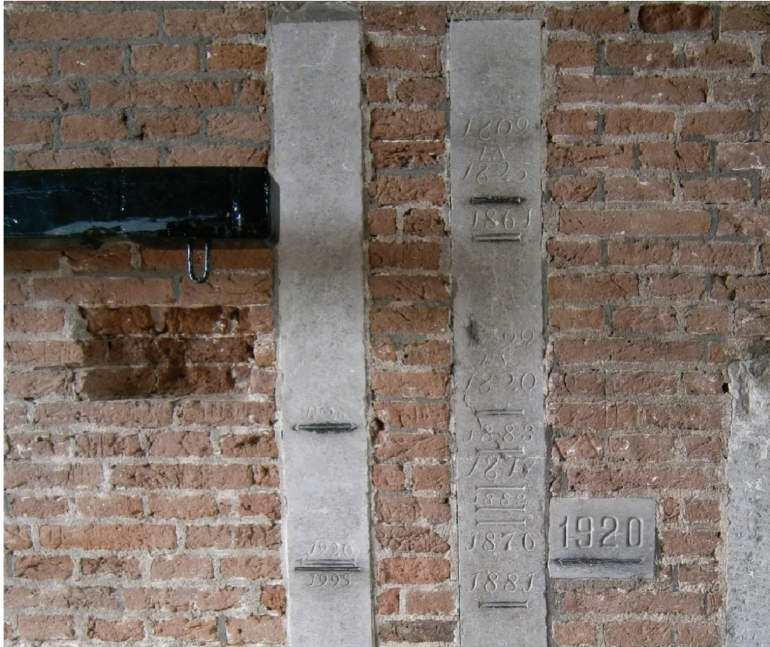
Figure 2.2: Flood marks at Slot Loevestein, the Netherlands [image credit Jan Tilma] approximate brick width 200mm
