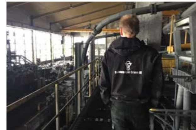
The Sydvaranger processing plant in Kirkenes. Photo: Ales Strøm
