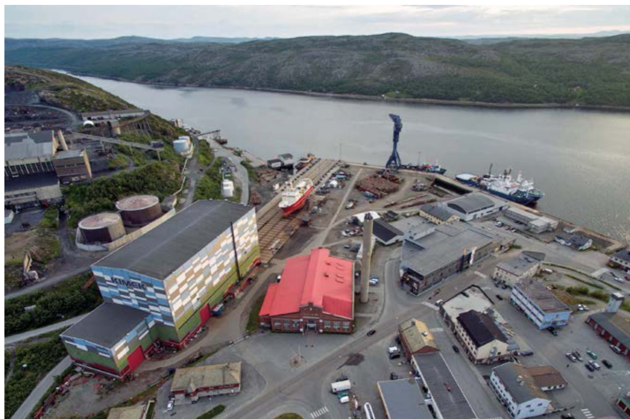
▲ Photo / 36 The KIMEK Drydock as new "landmark" of Kirkenes / Höller
