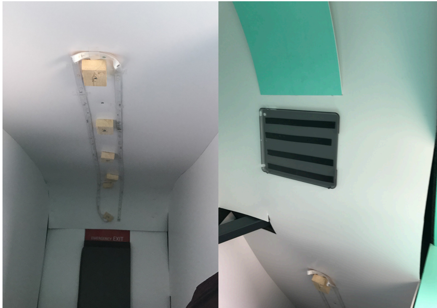
After integration of the LED strips it was needed to test them. As can be seen, they were working fine. The next step was to remove all the protection foil and to get the lower ceiling integrated. Not to forget, detailing. The control panel needs to be attached, as well as the rotation knobs. The first steps are displayed below.
