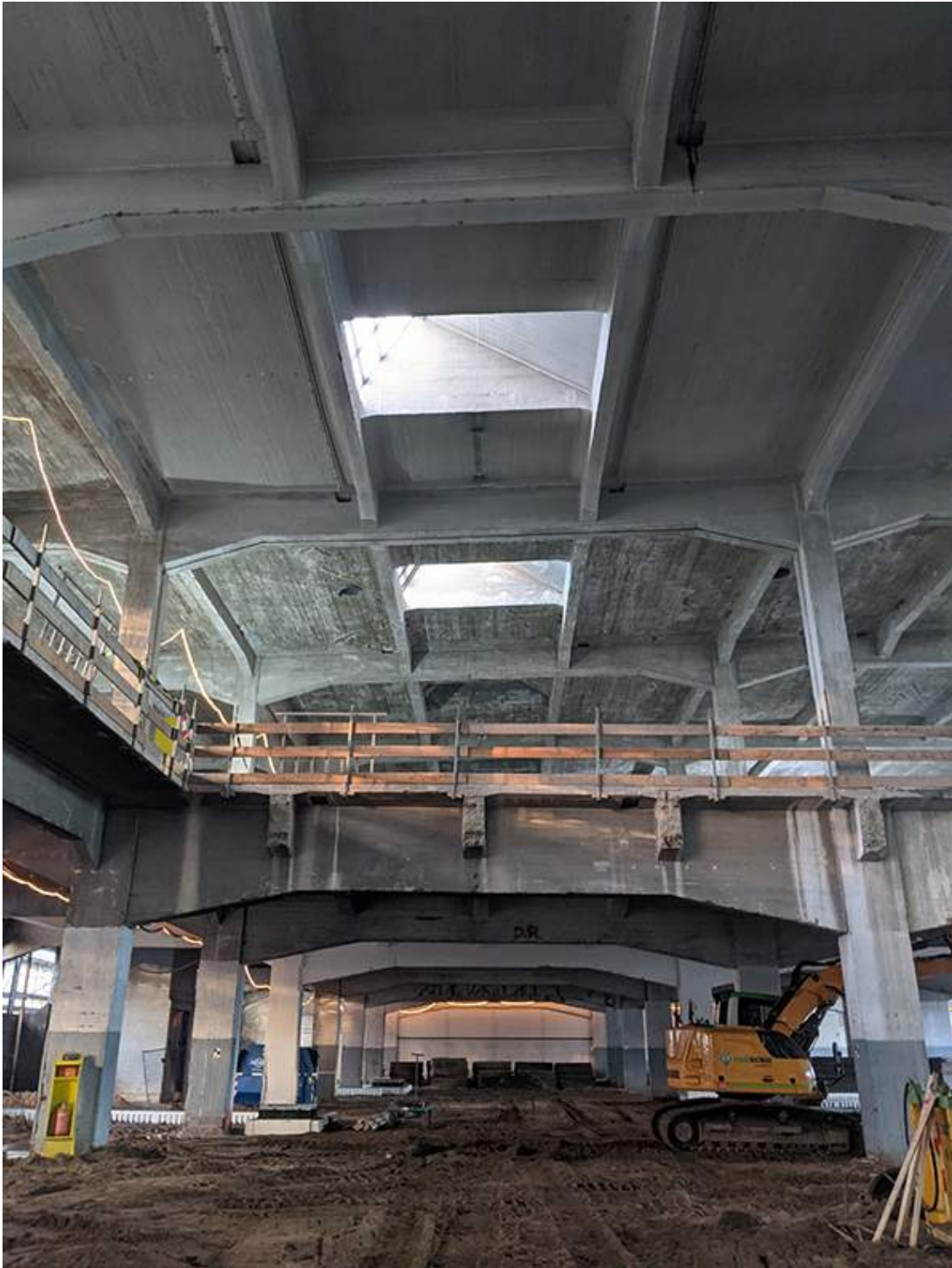
Fig. 5.9: Fenix II: ground floor looking west, 1916 construction
