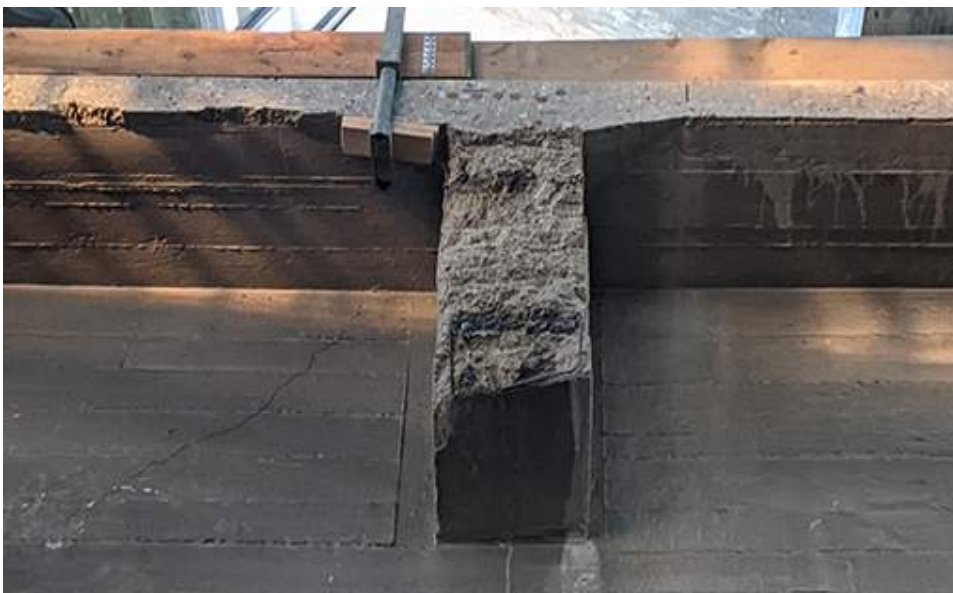
Fig. 5.13: Reinforcement at cut beam at Fenix II
