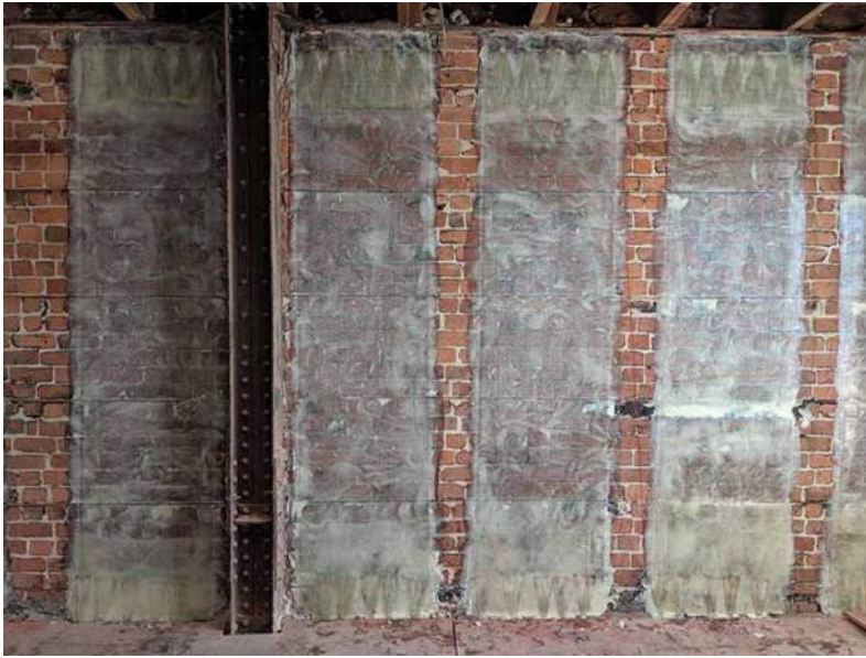
Fig. 3.4: GFRP by Simpson Strong-Tie bonded to a URM wall
