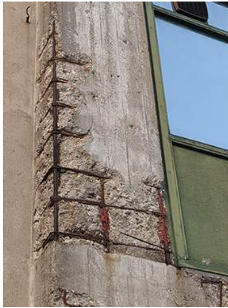
(b) East facade column
