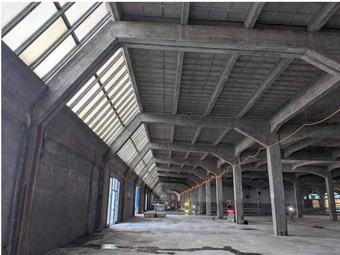
Fig. 5.11: Fenix II: first floor looking east, 1949 construction
