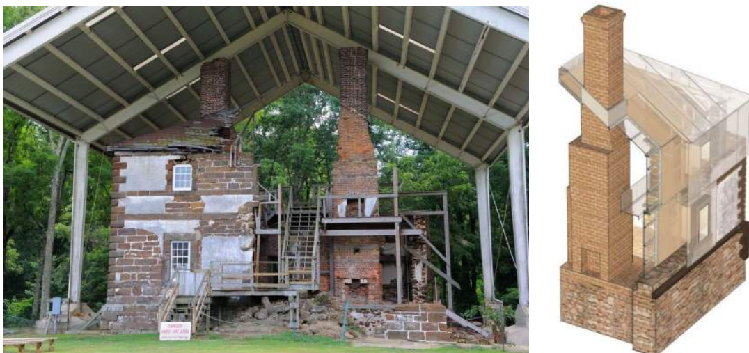
Fig. 4.13: Menokin House, US - Left: ruins in current condition; Right: section axon by Machado Silvetti
