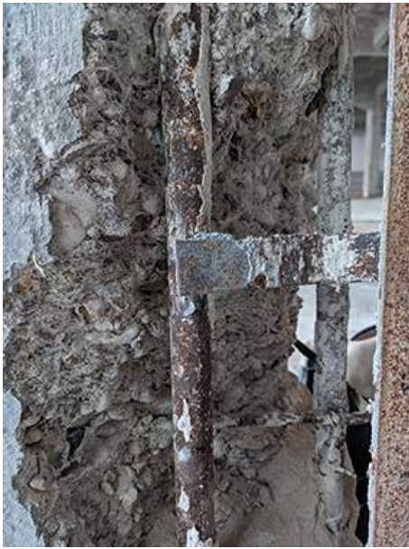
(a) Level 1 interior column
