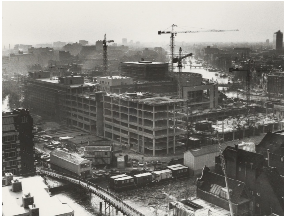
Figure 16 | The Stopera under construction (Source: Amsterdam city archive, 1985)
