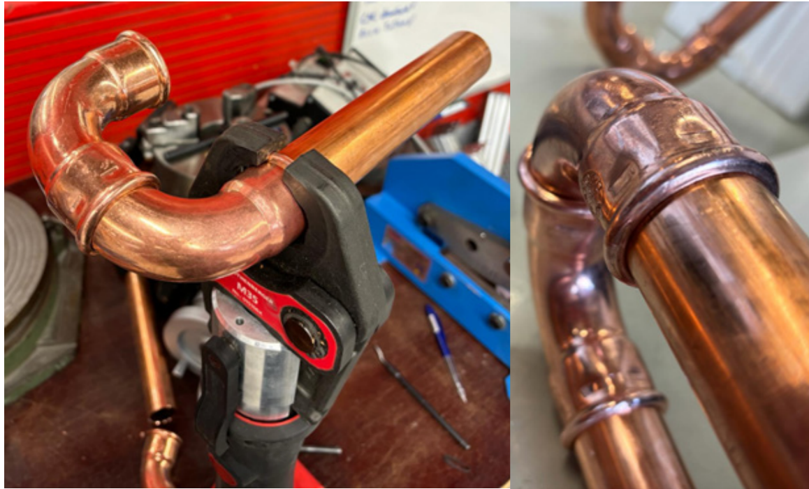
Attaching the bends and straight tube parts with a jaw press:
