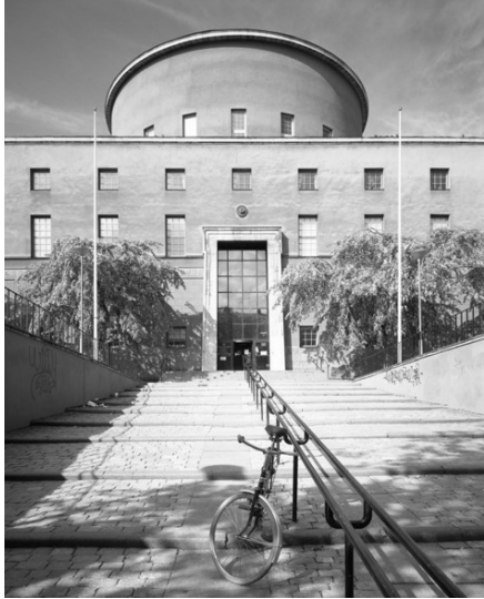
(Descending): Fig. 24. Stockholm City Library entrance portal, RIBA archival photograph (1987), Chris Martin; Fig. 25. Stockholm City Library entrance portal analysis, Sketch, NTS.
