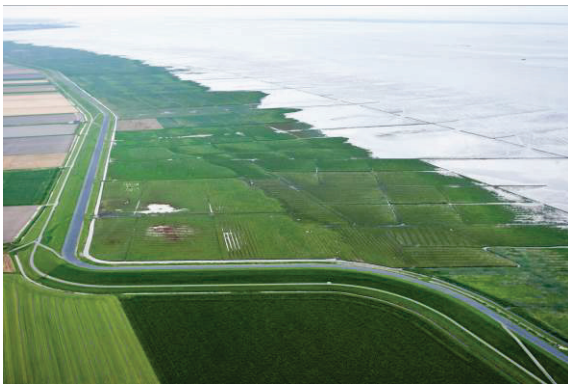
Groningen, salt marsh, Wadden Sea Marsh elevation 2.0 m+NAP, width 800 m, slope 1:750 Dike height 9.1 m+NAP, slope 1:4 Design conditions: h = 5.3 m+NAP, H_{m0} = 1.8 m, T_{m-1,0} = 5 s
