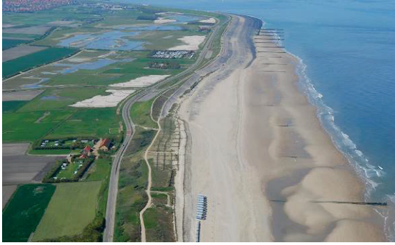
Westkapelle, sandy foreshore, North Sea Foreshore elevation 4.0 m+NAP, slope 1:40 Dike height 12.6 m+NAP, slope 1:6 Design conditions: h = 4.9 m+NAP, H_{m0} = 4.6 m, T_{m-1,0} = 9 s
