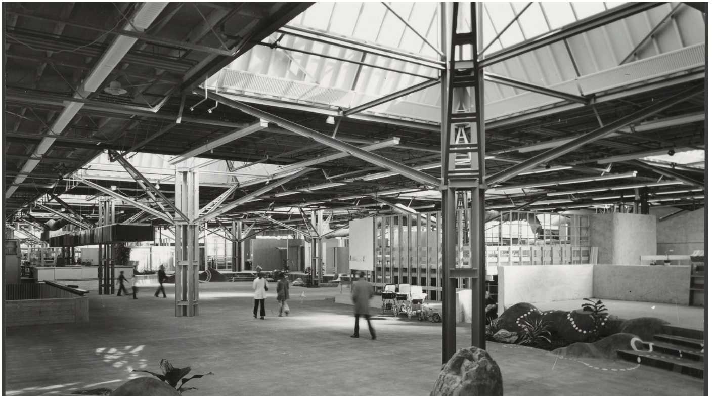
Image 7: Photograph of 't Karregat showing the structural tree like elements that made up the scheme of the building (1980-1985). Source: Het Nieuwe Instituut [photographer unknown]
