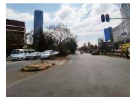
Road Surface Material:
