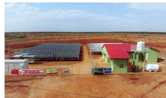
Figure 118: Photo of power station in Qorile village, Somali region of Ethiopia Source: Courtesy of CET, 2020
