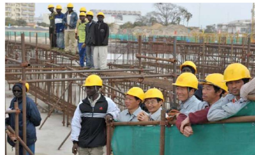
Figure 6: Senegalese and Chinese workers at the construction site Source: foreignpolicy.com/
