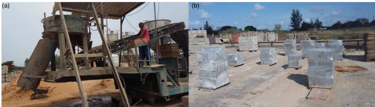
Figure 2 | (a) The equipment used to mix and mold the M15 concrete blocks. (b) The blocks wrapped in plastic to keep the moisture.
