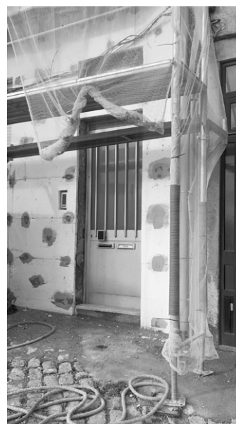
Renovation (own work)
