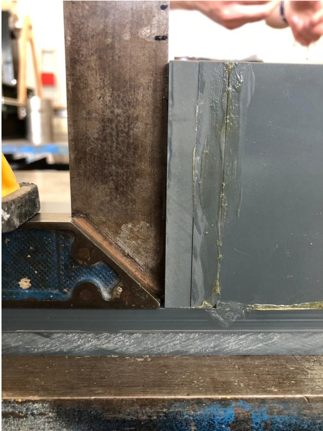
Figure 53: When gluing the horizontal overhang plate in to place, the angle of the overhang must be 90 degrees over the whole width of the tank.
