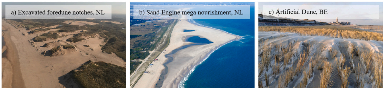
Fig. 1. Three dune intervention projects, having varying objectives. (a) Five notches in the foredune at the National Park Zuid-Kennemerland (NPZK) purposefully excavated to reintroduce dune dynamics. (b) The 21 Mm 3 Sand Engine mega nourishment, constructed to stimulate dune development. (c) An artificial dune constructed in front of an existing seawall as part of the Dune-in-front-of-Dike project to limit sand nuisance.
