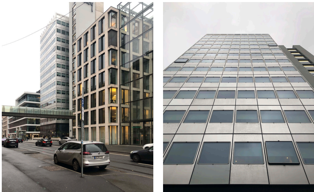
FIG. 6 The former Commerzbank high-rise after the recent upgrade and conversion, 21.11.2021. Photos: Rouven Grom
