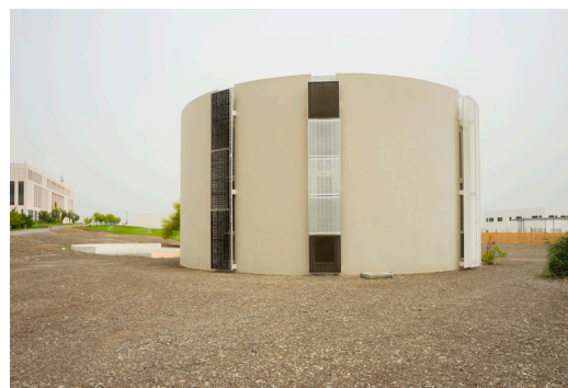
FIG. 6 Application of the passive ADAPTEX sun shading to the EcoHouse at GUtech in Muscat, Oman
