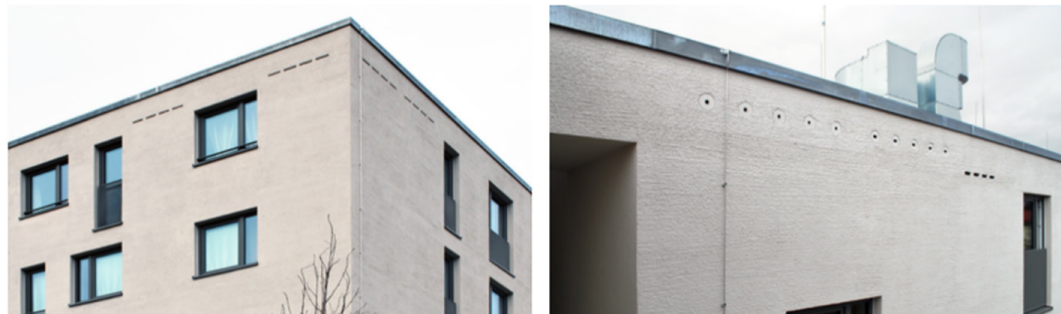
FIG. 2 Integration of nests into buildings' facades, Weisser & Hauck, bogevischs buero architects, 2015.
