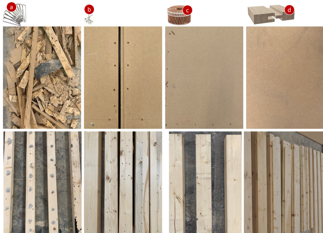
FIG. 6 OSB panels and wood mullions after the disassembly activity. The tests were carried out for four different connections between façade layers (a) staples and nails, (b) screws, (c) timber nails, and (d) interlockings. Images by the author.
