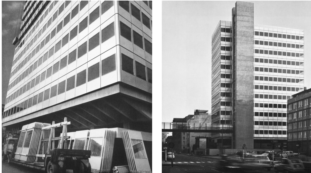
FIG. 2 The Commerzbank high-rise in Düsseldorf of 1962 by Paul Schneider-Esleben. Photos in Calendar Josef Gartner GmbH, 1963 April 21.-27. (left) + May 19.-25. (right). Photos: Inge Goertz-Bauer. Gartner archives, Gundelfingen (Donau)
