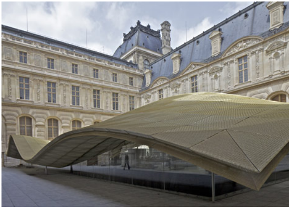
Figure 3.5: Example of free form architecture: Side view of Department of Islamic Arts at Musée du Louvre. Source from: [11]
