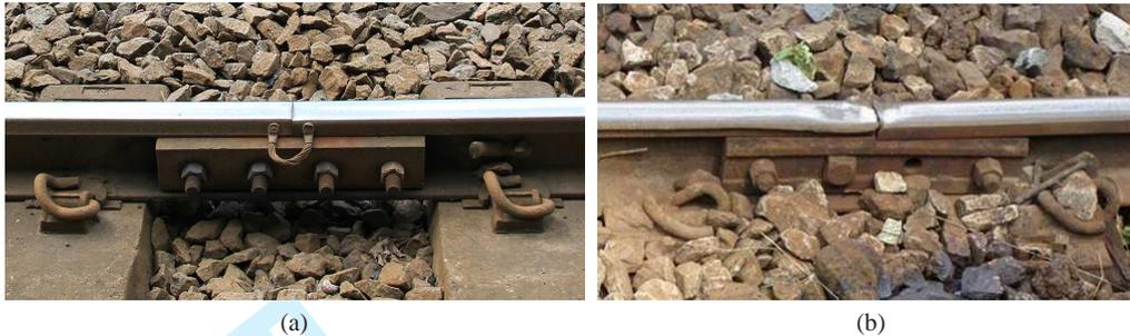
Figure 1. Two examples of rail joints: (a) invisible damage: loose bolts, and (b) visible damage: missing bolt and battered rail surface
