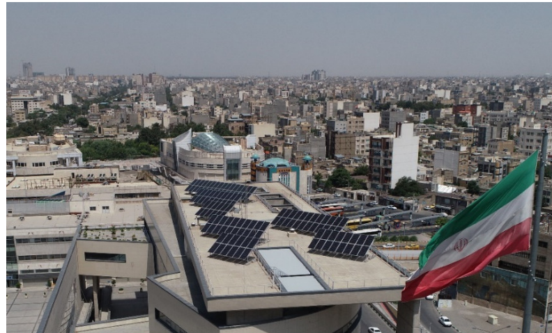
Figure 6. Aerial view of the 51 kW GCPVS on the Mashhad City Hall building.
