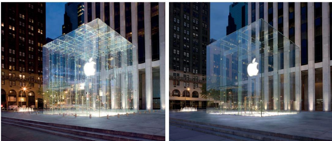
Figure 1.2: 5th Avenue Apple store in New York built in 2006 (left) and 2011 (right)
