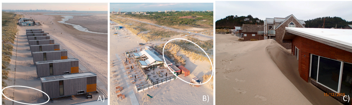
Fig. 1. Buildings on the beach. A) A row of holiday houses with some deposition behind the houses (e.g. the white oval), in Kijkduin, The Netherlands. B) A beach restaurant with a more bare dune behind it (the white oval) in Kijkduin, The Netherlands. C) Houses with substantial deposition built in Pacific City, USA (photo courtesy of Oregon Parks and Recreation Department).
