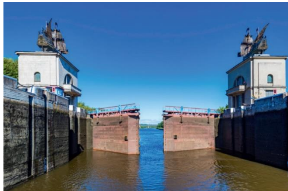
Figure 72: Mitre lock gates, source: (Allianz)
