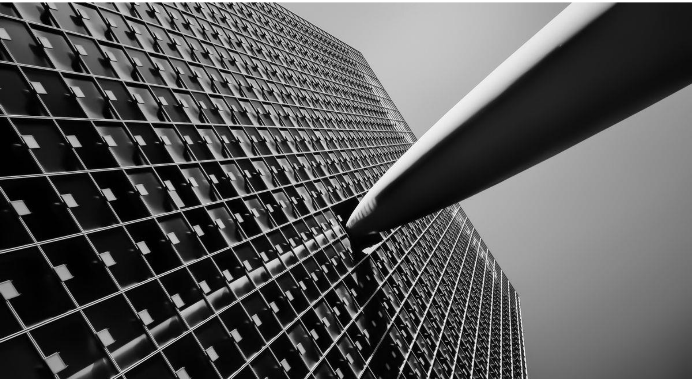
“KPN Telecom Toren” – Rotterdam
