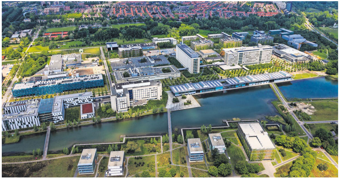
Figure 2.9 (top) The TU Delft campus with buildings on a site of 161 hectares
