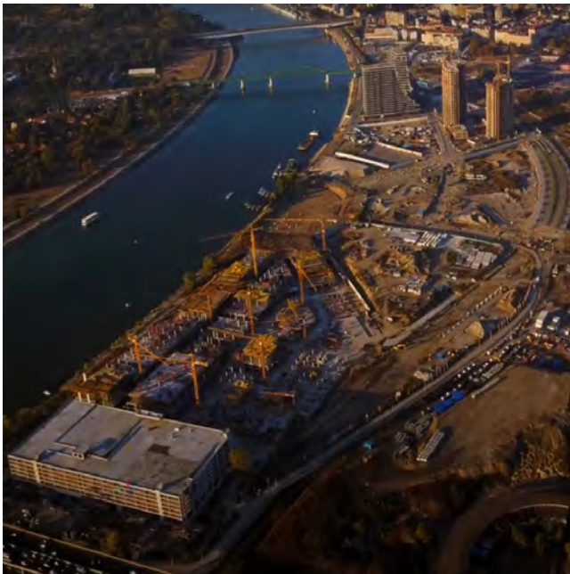
FIG. 4.8 Belgrade Waterfront - construction site, source: https://www.youtube.com/watch?v=WfLR0-H_EHE
