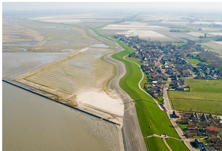
Figure 2.10: Vegetated foreshore, Friesland (beeldbank.rws.nl)
