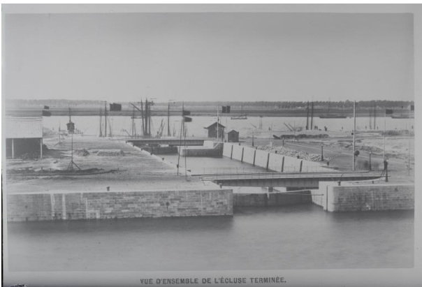
the lock and part of the docks in ca. 1920
