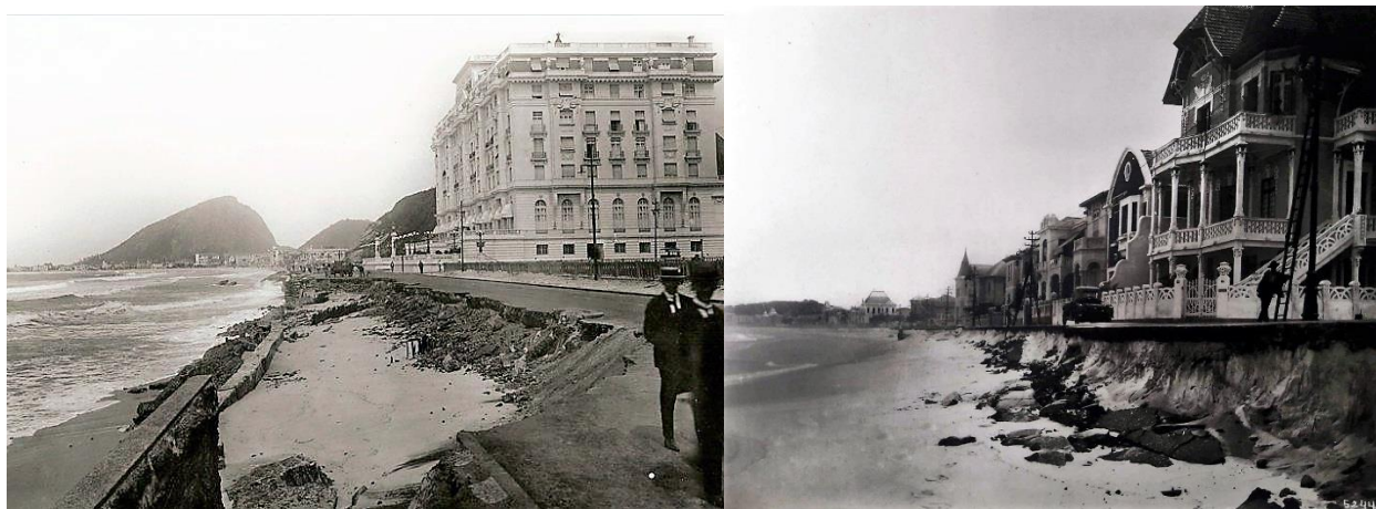
Figure 7: Two historical pictures showing damage due to wave impact on Copacabana beach in the 1920s (Lins-de-Barros et al., 2019).
