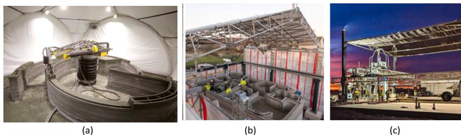
Fig. 14. On-site control and/or mitigation of environmental conditions during printing via a) complete enclosure [138], b) partial enclosure [139] or c) roof cover only [140].
