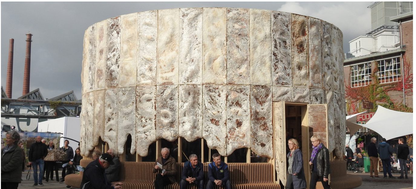
Figure 3: A pavilion with the facade panels grown using Mycelium, Pascal Leboucq and Krown Design.
