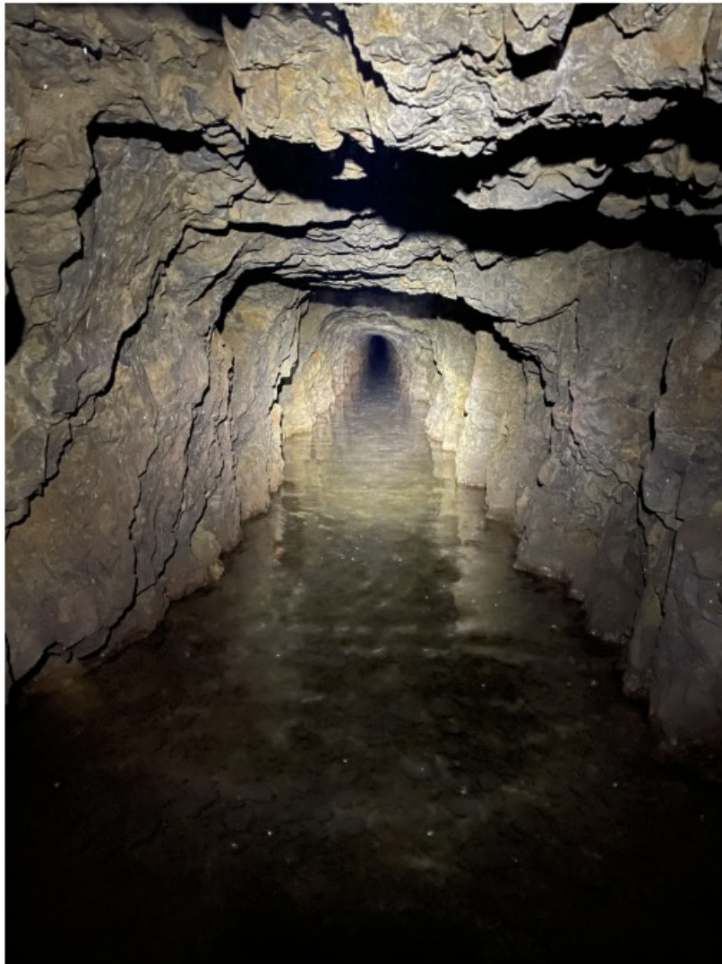
Figure 4.7: Dolomeuse Gallery, 1.5m wide. The shafts have been excavated at a pace of 1-3m a day (Pacyna & Denayer, 2010)
