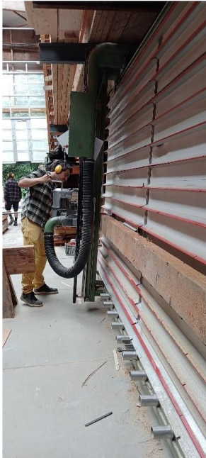
USING THE VERTICAL WALL SAWY TO CUT THE PIECES
