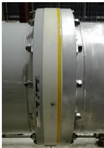
Figure 3. Spacer and flanges joined with bolts.
