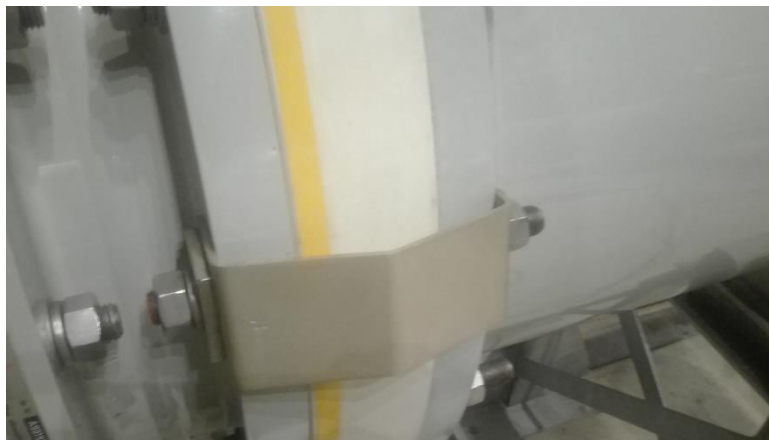
Figure 39. Bridge between to flanges.
