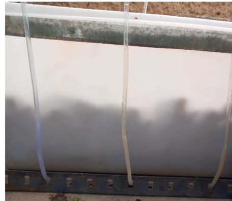
c Piezometers installed for controlling the water level
