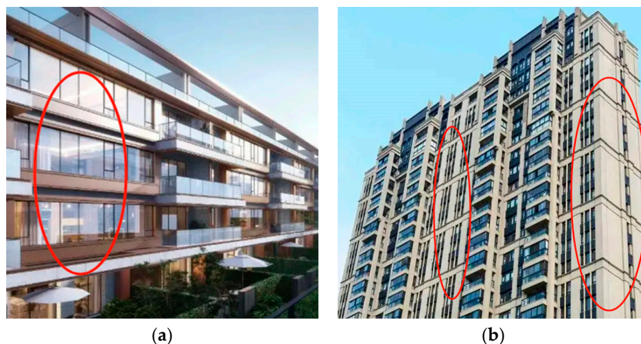
Figure 1. Exterior building fire protection component. (a) Eaves case. ( https://www.sohu.com/a/771292546_121342467 , accessed on 5 May 2024); (b) Partition bands case. ( https://co.pinterest.com/pin/351914158382391979/ , accessed on 5 May 2024).
