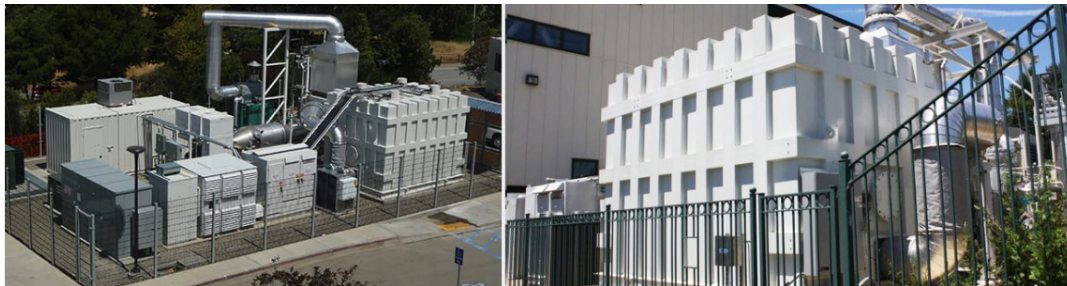
Figure 6.5: SureSource1500 by Fuel Cell Energy (Fuel Cell Energy, 2022 ).
